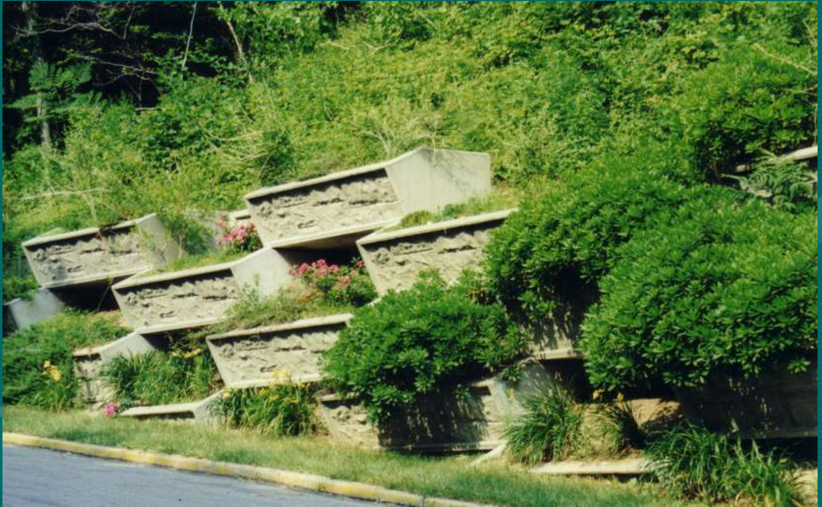
Evergreen GEO wall after one year
