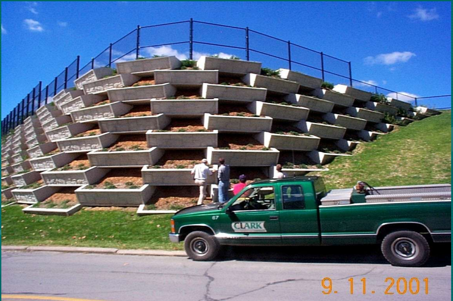
Final Check of Construction
