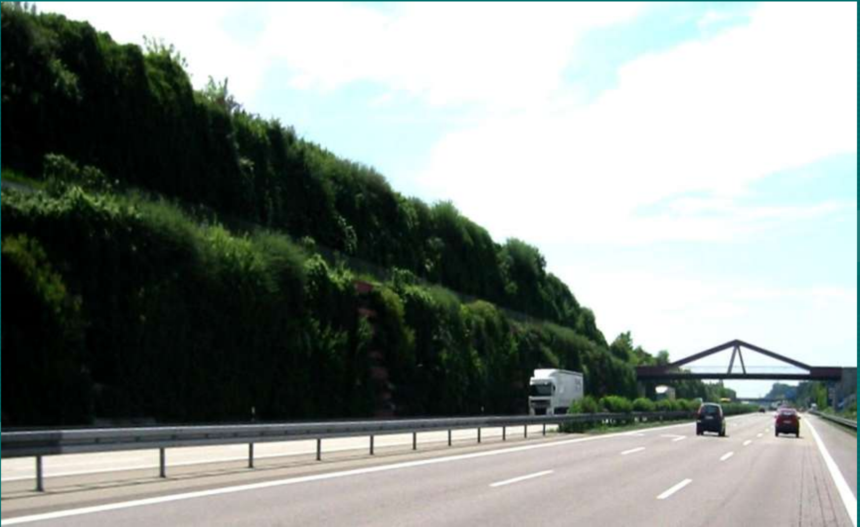
Evergeen GEO near Karlsruhe, Germany
