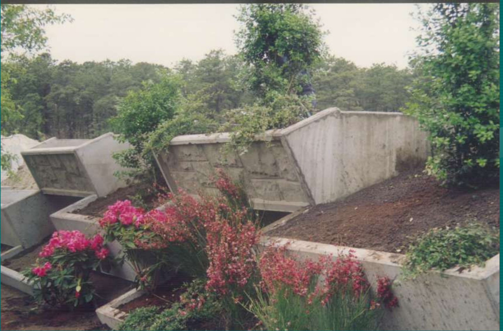
Evergreen GEO Wall, Brookhaven, NY, USA
