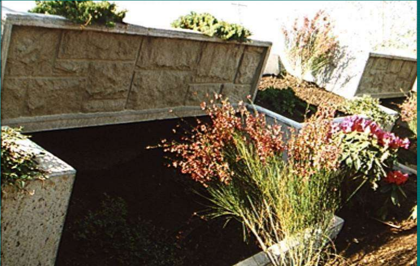
Planted Evergreen GEO Units
